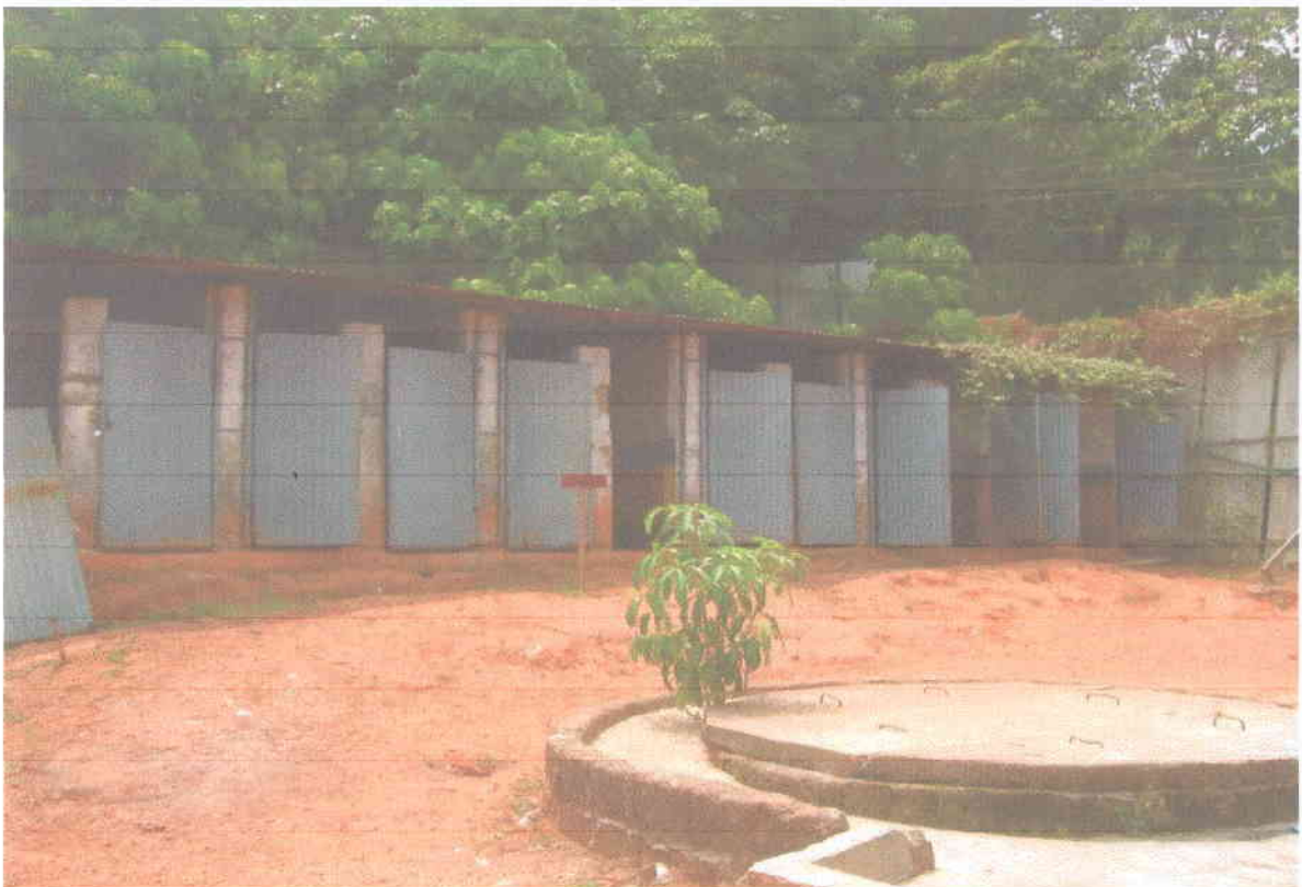
PHOT. 3 Toilet facilities in labor camp
