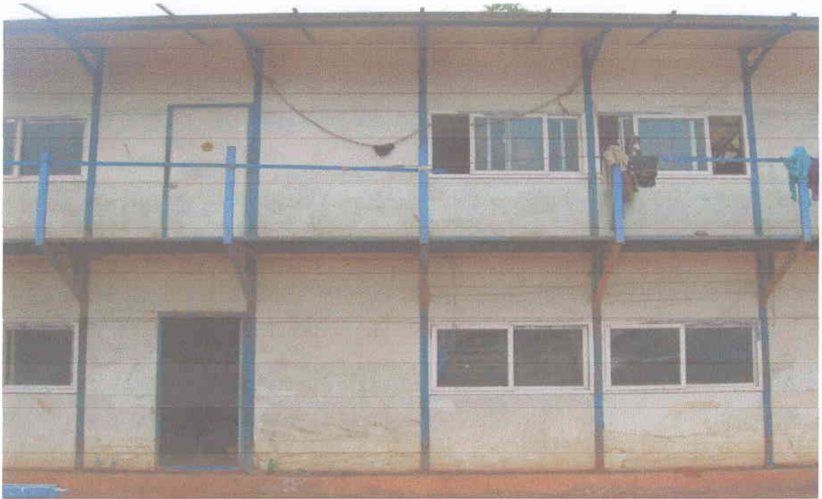
PHOT. 2 Temporary Labor camp – near to the site residing 100- 120 labors
